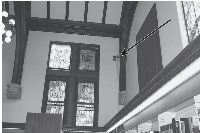
FIGURE F.4(c) Linear Beam Smoke Detector.
