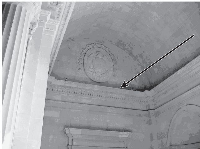
FIGURE F.3(c) Exposed Sprinkler Pipe.
