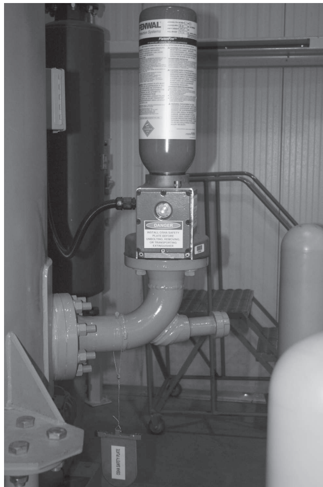
FIGURE 6.2.3.6.1.2(a) HRD Suppressor with 75 mm HRD Valve.
