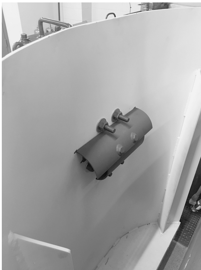
Δ FIGURE A.5.2.5.2.1(b) Foam Chamber Deflector.
