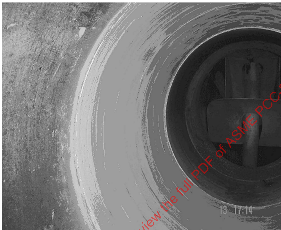
Figure 403-1.1-1 Structural Liner in Raw Water System
