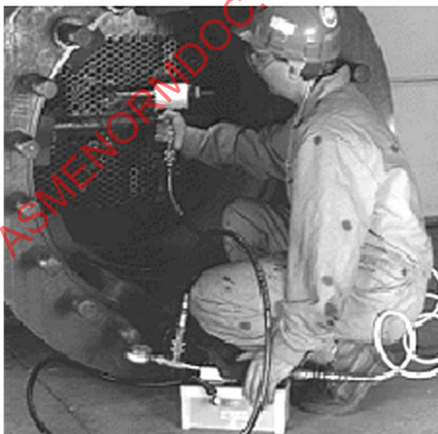
Figure 312-4.2-3 Typical Installation of Mechanical Fit Tube Plugs
